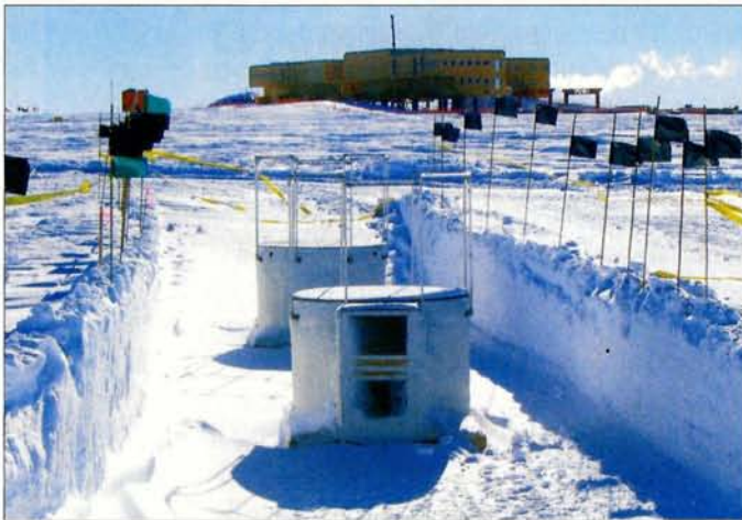
Fig. 4. Two IceTop tanks being installed in a shallow trench.
